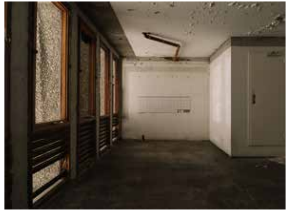
Interior photo from H-Block
